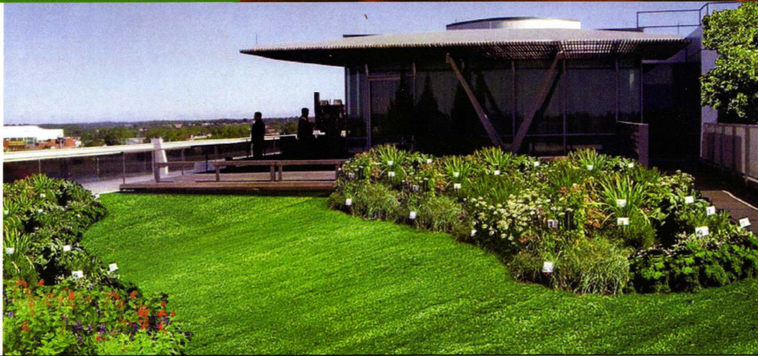
Tremco green roof assembly installed over Clinton Library. In 2007 the Clinton Library and Museum received its LEED Platinum certification.
