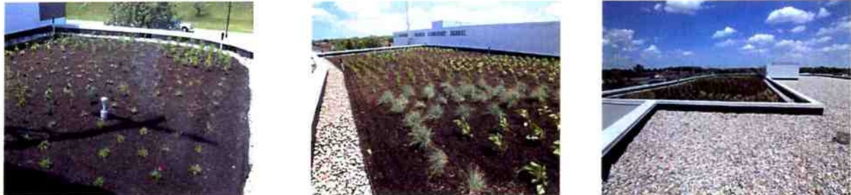
View of plant materials after installation by Landscape Effects
