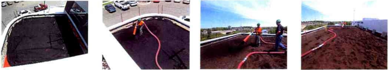
Blowing of soil conducted by LandSource Organix Ltd
