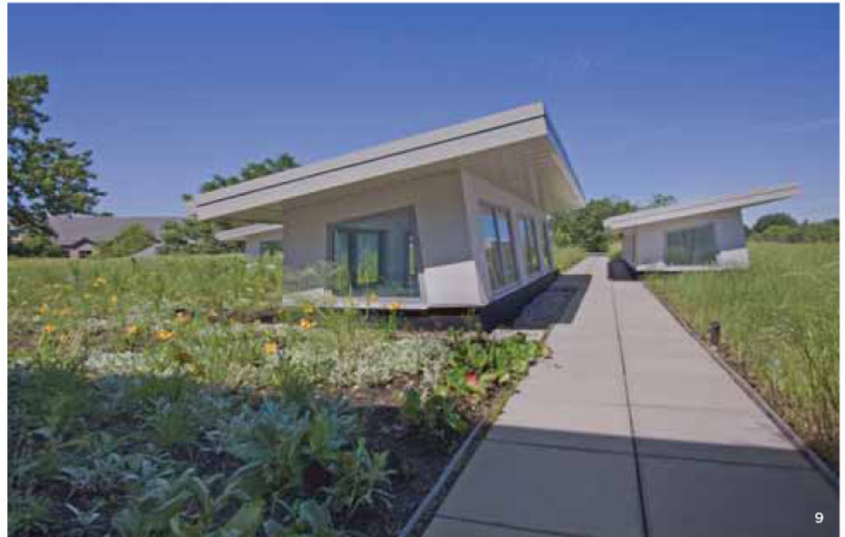
ROOF-TOP MONITORS ON THE GREEN ROOF BRING NATURAL LIGHT INTO THE CORE OF THE BUILDING [9].
